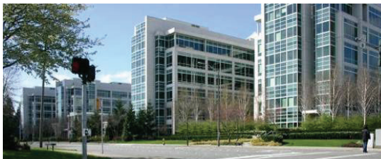
Microsoft plans to add 2.2 million square feet for 12,000 additional employees within the next several years. To support this growth, Microsoft will be completing approximately $35 million in street and sewer improvements, including the new SR 520 overpass connecting NE 31 st to NE 36 th Street
